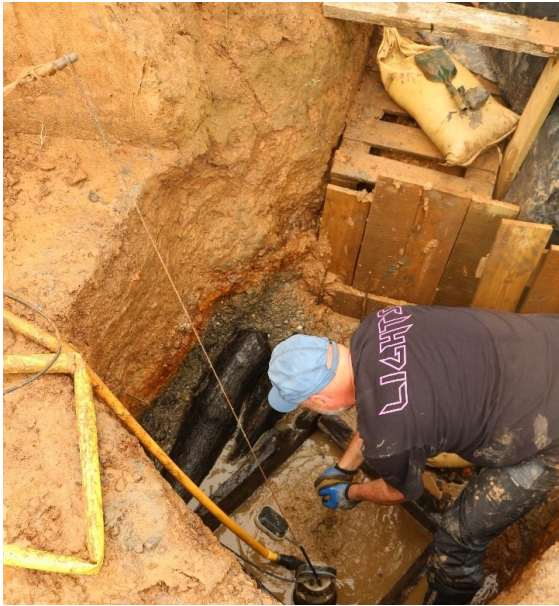
8.72: Excavation was cramped by the protective shuttering and waterlogged despite pumping
